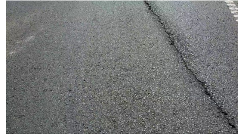
D3. Unconnected crack that typically cuts across the road in a diagonal direction.
