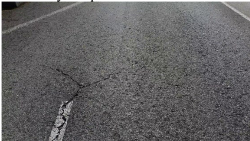
D5. Unconnected cracking with non-defined geometry.
