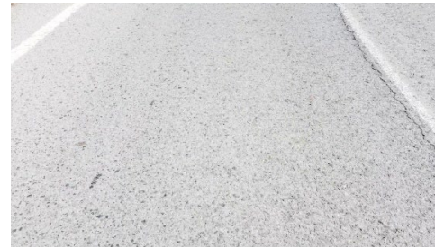
D7. Same as longitudinal cracking but between lanes.
