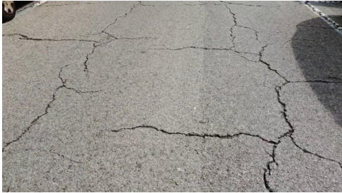
D1. A sequence of interconnected blocks, essentially rectangular in shape, are created by the pavement's entire surface.
