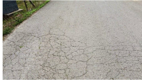
D2. Interlaced fractures that typically, generating a succession of tiny polygons like the crocodile hide.
