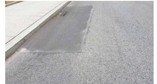
D8. Portion of pavement that has been removed and replaced.
