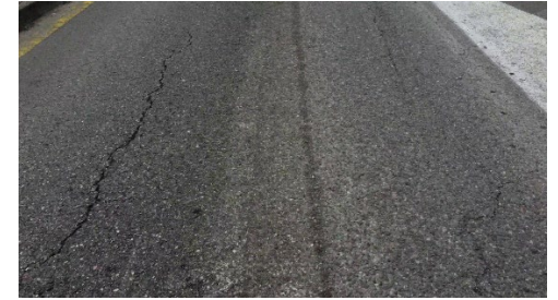
D4. Unconnected longitudinal crack present in wheel/non-wheel paths.
