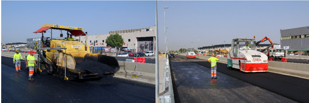
Figure 13. Laydown and compaction
